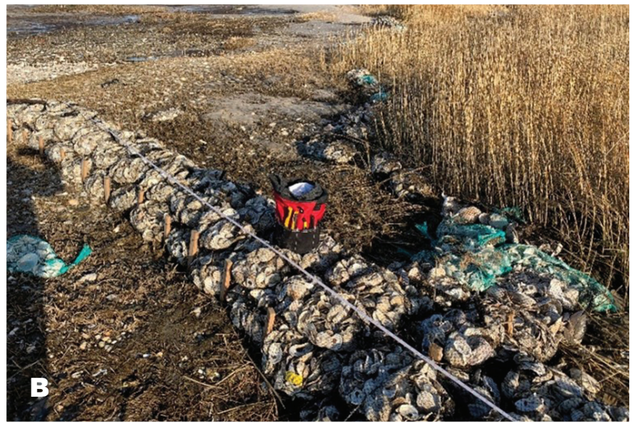
Figure 2 (above). Several creative solutions aided restoration of Gandy's Beach Preserve, New Jersey. (A) Rafts were designed and constructed to transport materials to their final deployment site. (B) Specialized stacking and anchoring of shell bags allowed their placement in higher energy environments than typical.
